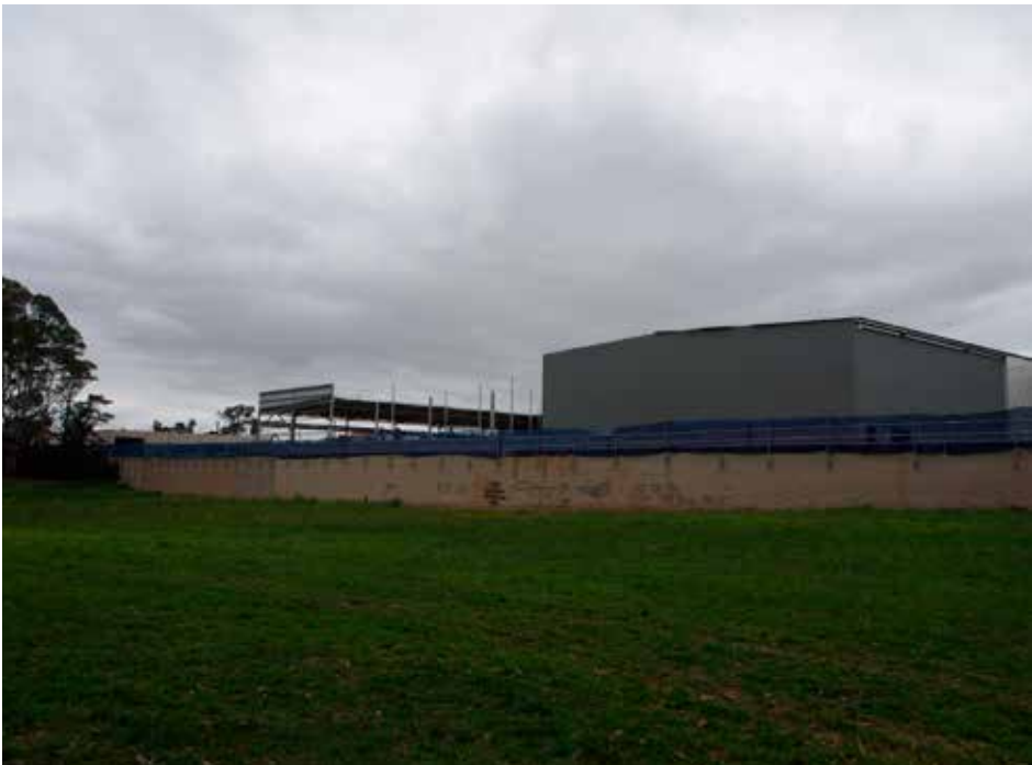
The Masters Home Improvement site under construction adjacent (west) to the site.
